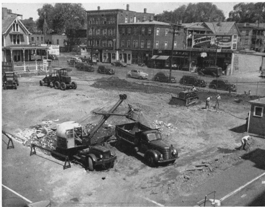
Getting its face listed is the Hayden Street parking area. Steam shovels and trucks are busy cleaning off the lot for re-surfacing. Other parking areas will be done in their turn, announced Chief John J. Bergin, Plant Protection. Notices will be posted in these areas before work begins to give all drivers time to find other parking spaces.
